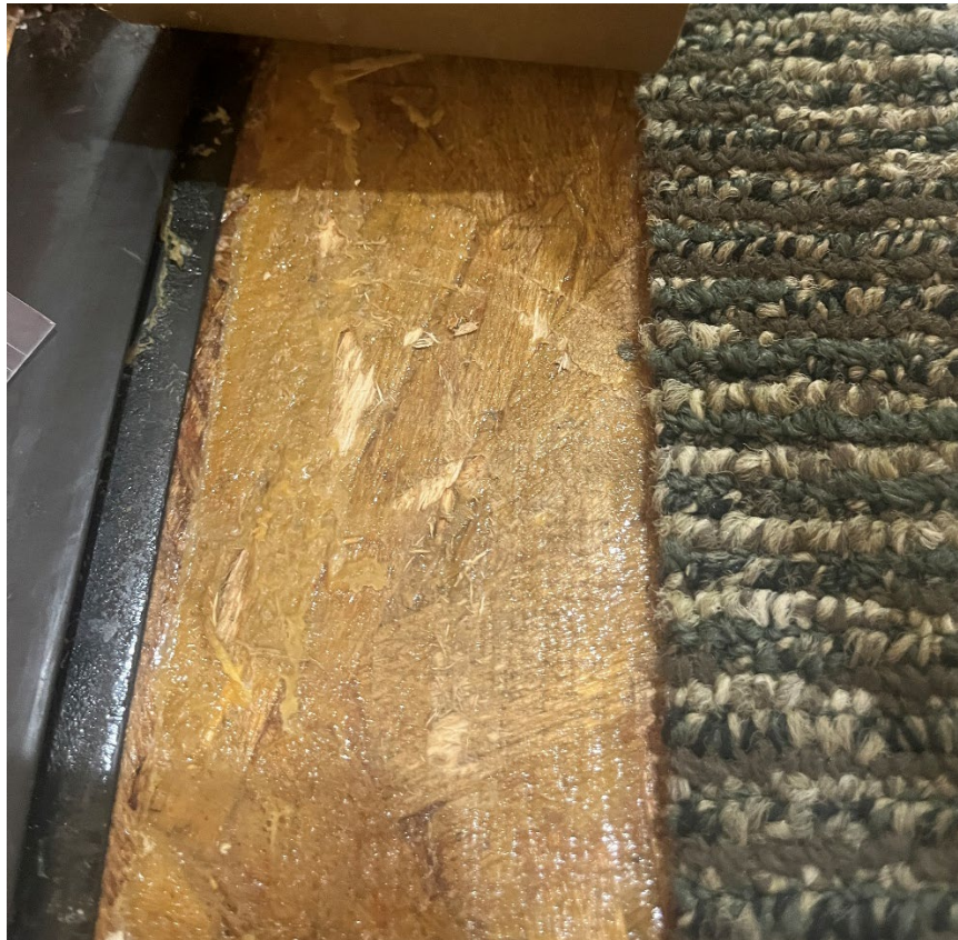
Photo 4: Non-ACM blue/gray carpet with associated tan mastic on plywood
