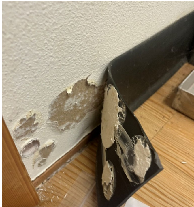
Photo 2: Non asbestos-containing (non-ACM) gypsum wallboard and dark gray cove base with associated yellow mastic.
