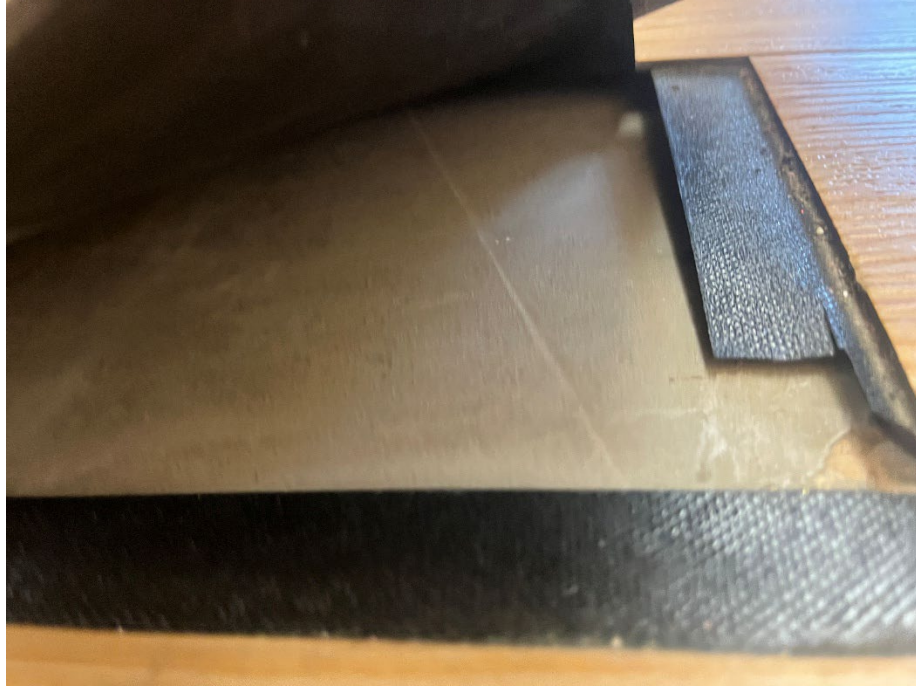
Photo 3: Non-ACM black adhesive tape under laminate flooring
